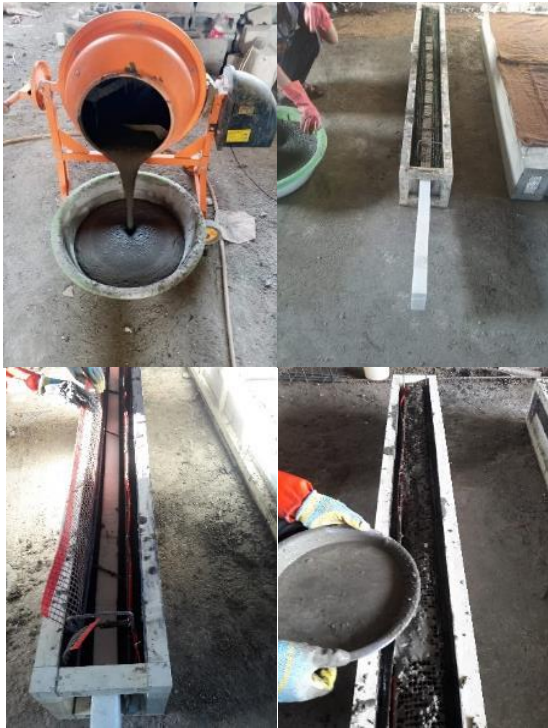
The casting of the beams using self-compacting mortar.
