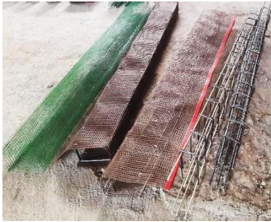
Beams reinforcement.
