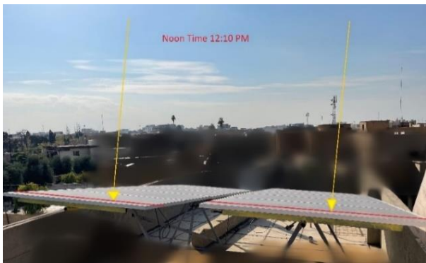
Fig. 3. Pv panels set in two rows and track the sun position at noon time.
