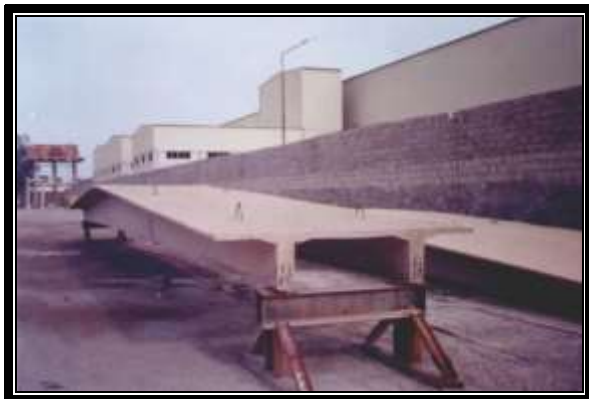
Fig. (11). Beam B2 – General view before testing.
