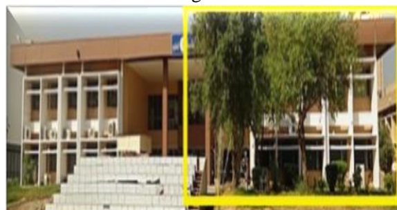
Figure 1. Dept. of Computer Science (CS) building – College of science - UoBaghdad (the case study)
