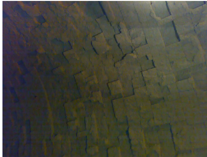
Fig 20 : Ovality (about 3 months of kiln operation ,Kufa cement plant, kiln No.2,tire base No.1) about 20% of brick thickness(4 cm) is fall down.
