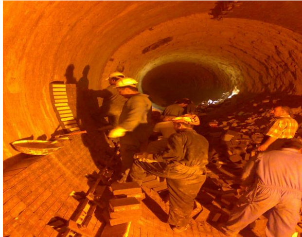
Fig 5 :Refractory Brick Re-building at Kufa Cement Factory (Kiln No.2).
