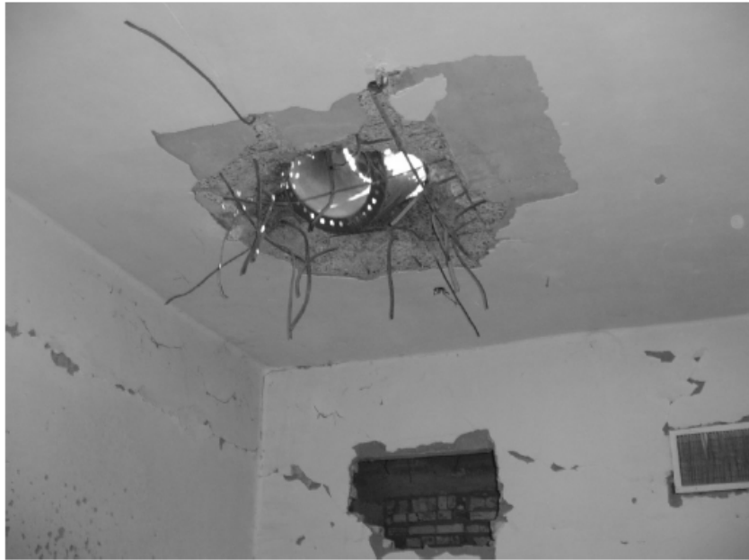
Fig. 1: Hole in the Reinforced Ceiling of the building
