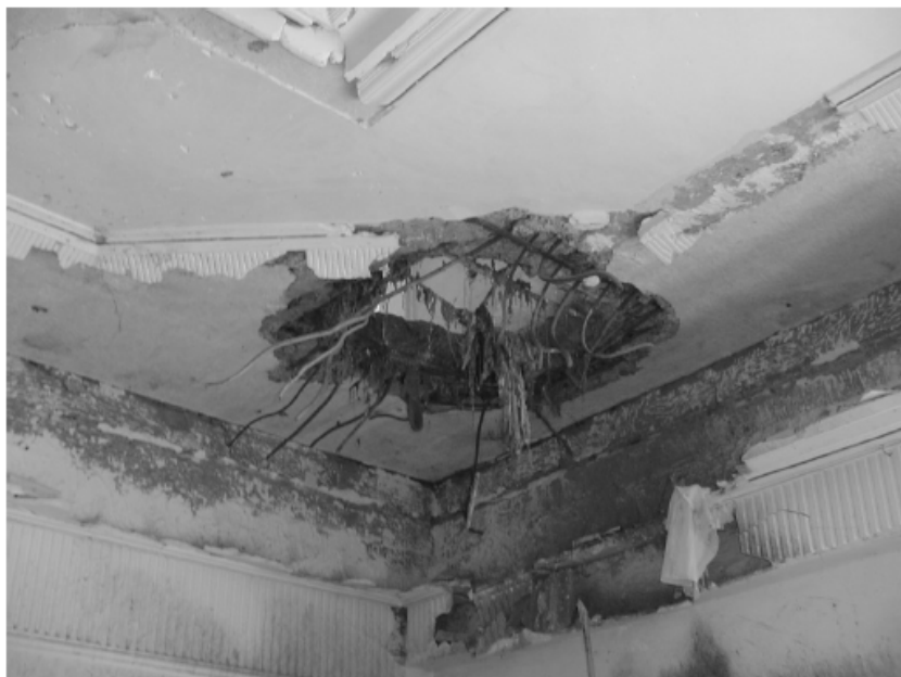
Fig. 1: Hole in the Reinforced Ceiling of the building
