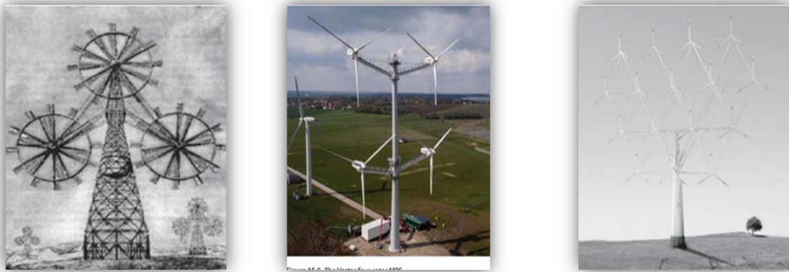
Figure 5: (a) Multi rotor by Hermann Honnef, 1930 [31], (b) Four rotor Array [33], (c) Rotor array [30]
