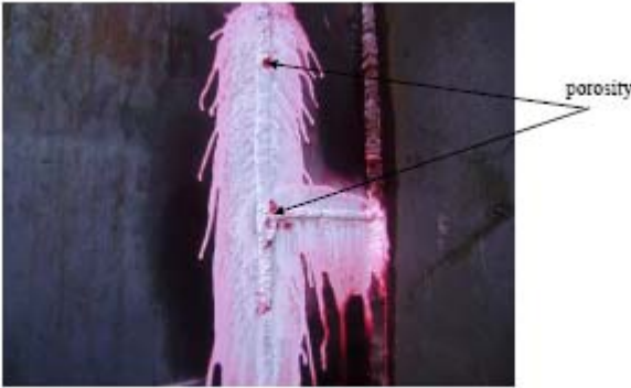
Fig ( 5 ) welding defects – porosity.
