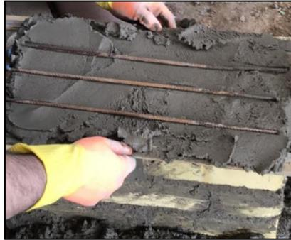
**Fig. 9. Utilization of steel reinforcement bar during erecting the fourth wall**
