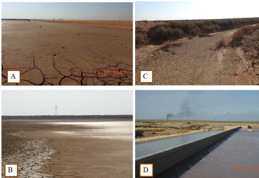
Fig.12 A , B show accumulation of silt in dry reservoir in January 2017 .C shows bed sediment of Dewerige river . D shows upstream & downstream of dam.
