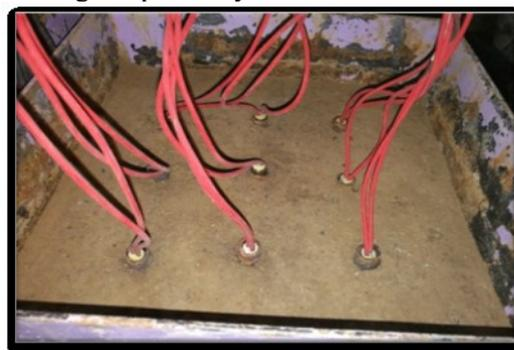
Figure 5: Electric heaters instillation
