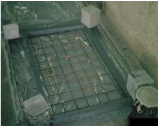
Fig 2 : Arrangement of steel reinforcement bars in the mould before casting.
