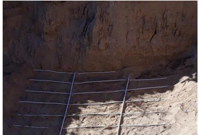
Fig. 3 MLCP pipes buried on depth 3 m.
