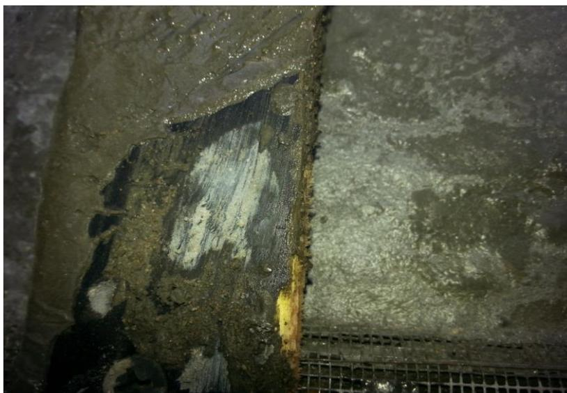
**Fig.(5). Fresh concrete permeated fiber wire mesh**
