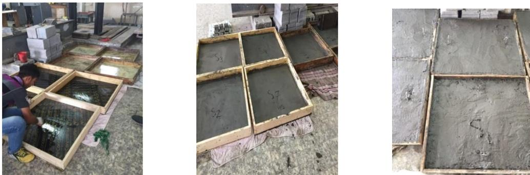
**Plate. 2: Concrete casting**
