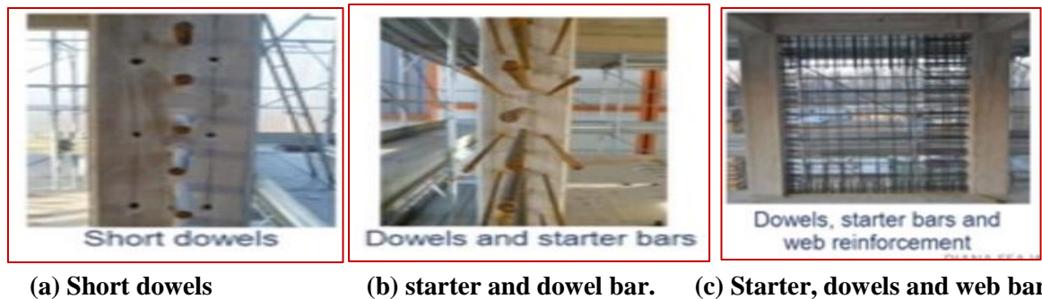
Figure 10. (a) Short dowels, (b) starter and dowels bar, (c) Starter, dowels and web bars
