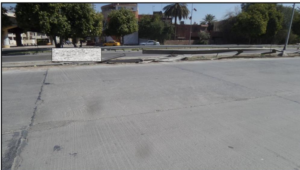
**a) Transverse Tining PCC pavement surface texture (Section No.1)**
