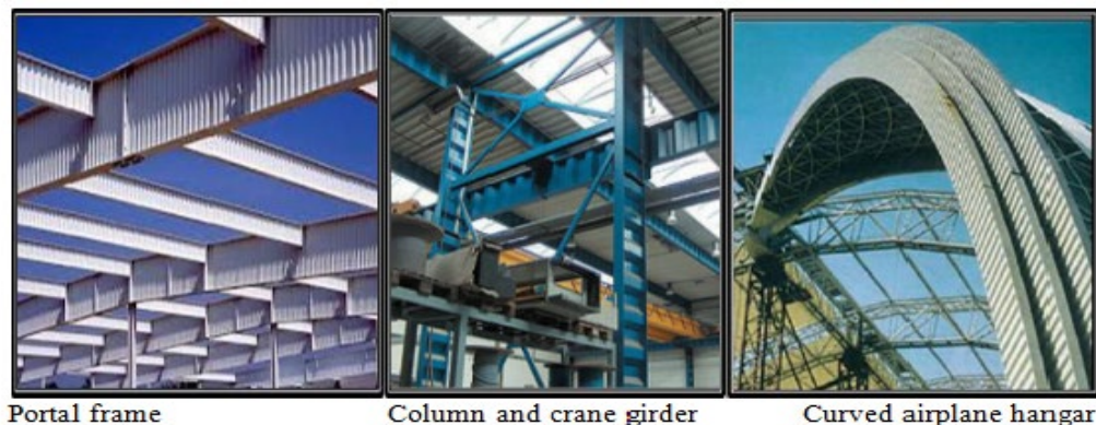
Figure 4: Corrugated web girder in industrial buildings
