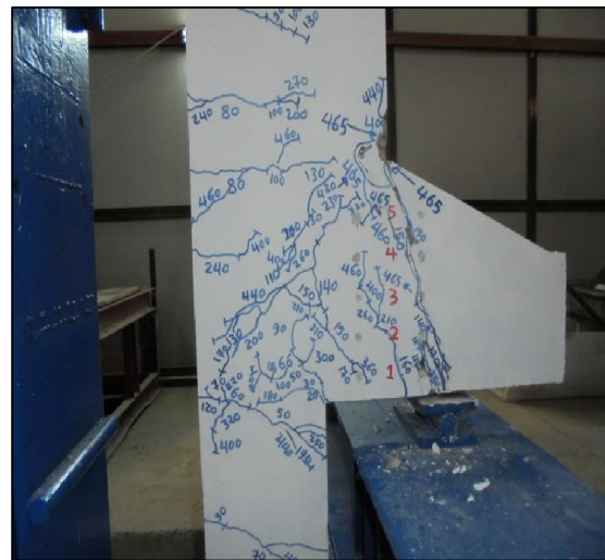
Fig.5 (b) Failure Mode of Specimen C2
