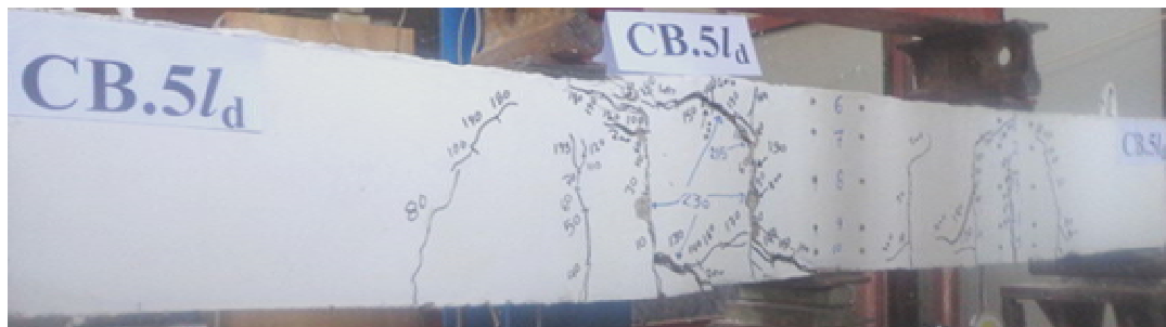
Fig. 11- Failure Mode of Girder CB.5l d
