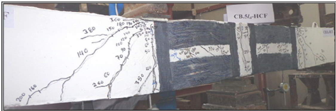
Fig. 15- Failure Mode of Girder CB.5I d -HCF
