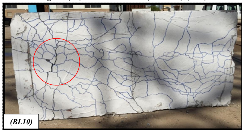
Figure (16): Crack Pattern ( D/t = 0.6 ) (BL10).
