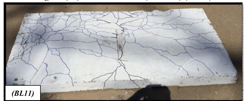
Figure (17): Crack Pattern ( D/t = 0.7 ) (BL11).
