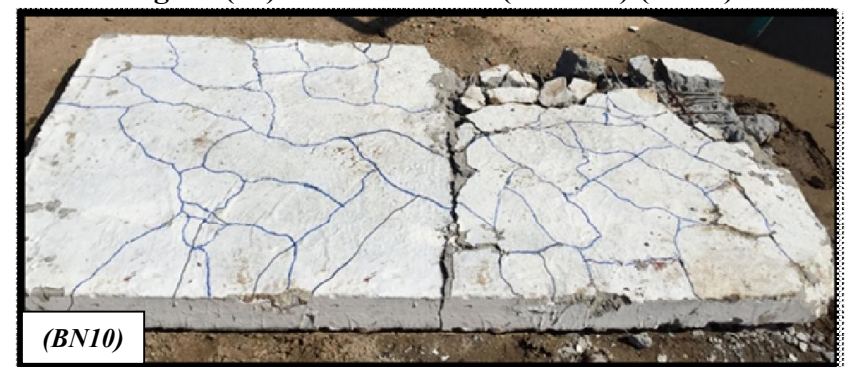
Figure (18): Crack Pattern ( D/t = 0.6 ) (BN10).
