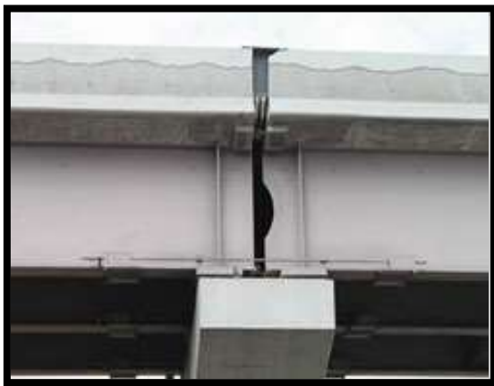
Figure (2): Steel bar restrainer
