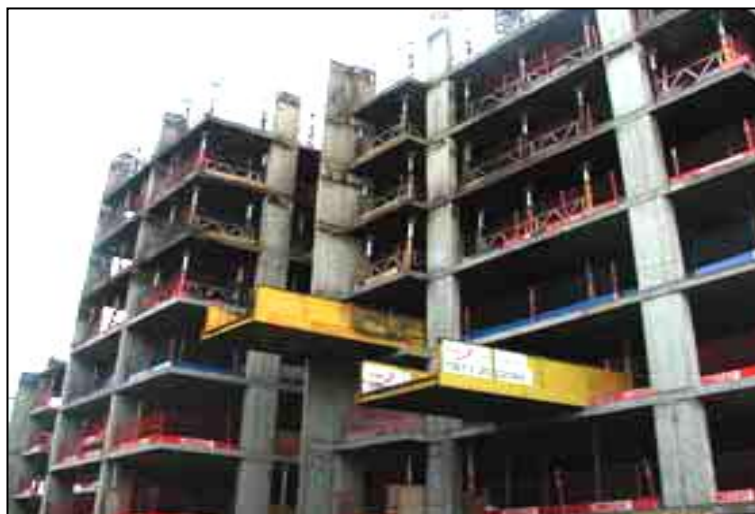
Plate (1): The concrete frame of a ten-storey building that was fire-damaged during construction, ( Ingham and Tarada, 2007).
