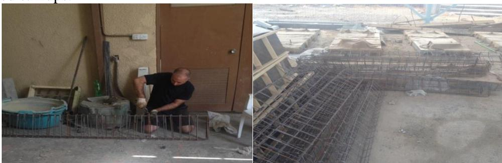
**Figure (17):** Cage of steel reinforcement.
