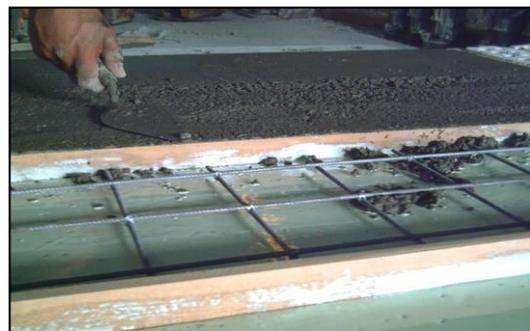
**(b): Casting of concrete overlay**
