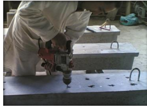
Figure 4: Process of the drilling
