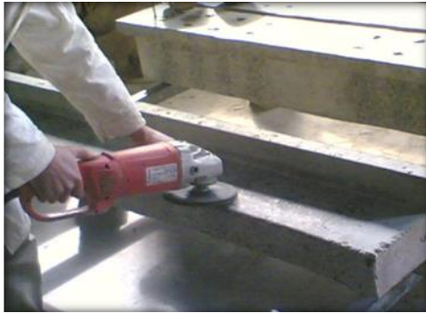
Figure 3: Concrete surface preparation by electrical grinder
