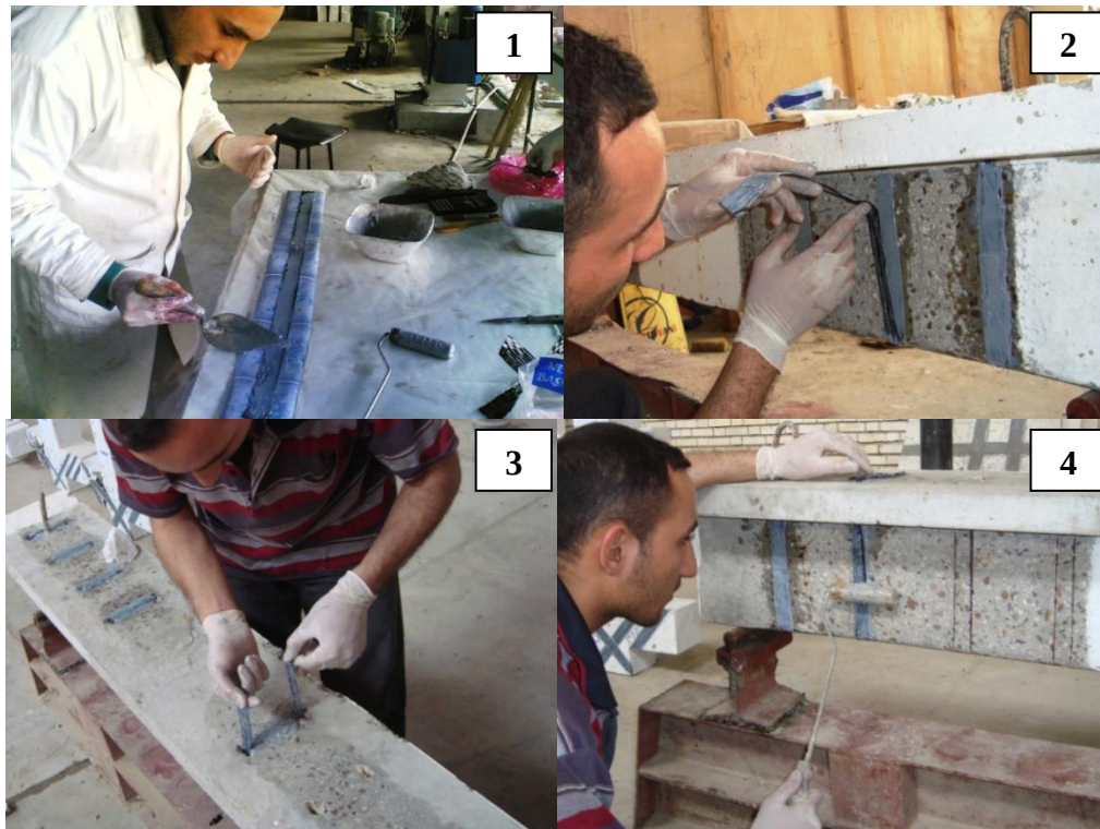
Figure 5: Application of CFRP sheets
