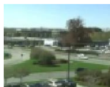
Reconstruct Frame 26th
