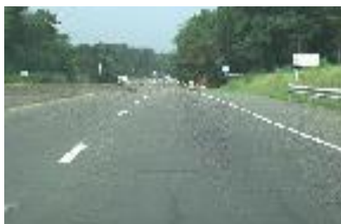
Reconstruct 26th Frame
