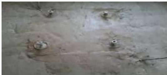
Figure 7: Preparation of a clay surface prior to connecting the pile cap to piles
