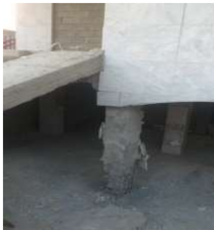
Plate 3 and 4: Column damage due to explosion.
