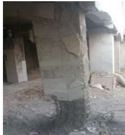
Plate 3 and 4: Column damage due to explosion.
