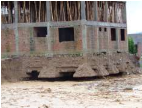
Plate 1: Soil erosion under Spread footing
