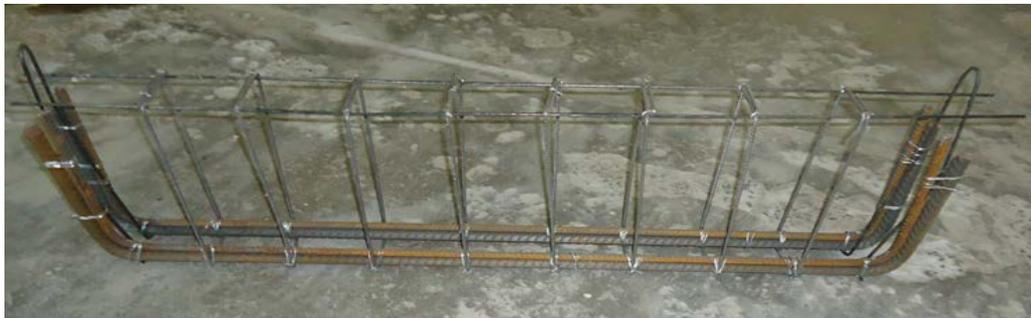
**Figure (3) Steel reinforcement cage used for beams construction**
