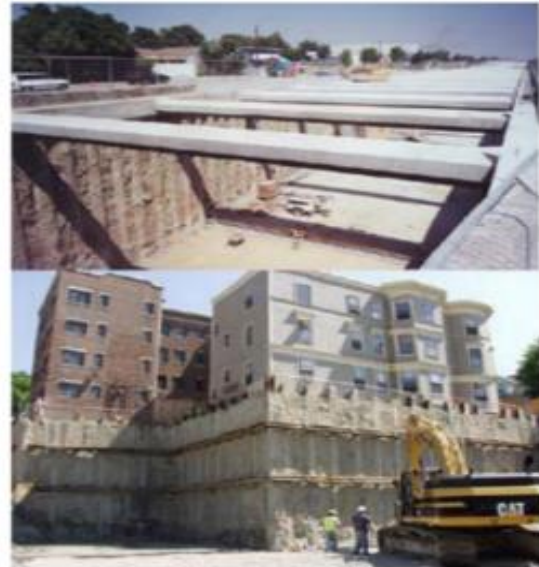
Figure 11. Above A railroad trench excavating job for the Alameda corridor. Bottom: A structural cutoff wall built during the building of a new Harvard University building in Cambridge[18]
