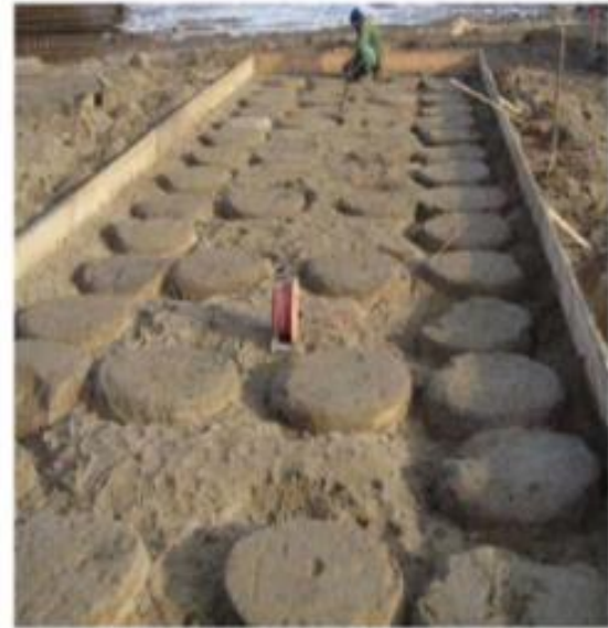
Figure 8. Foundation for Motorway Bridge near Katowice[18]
