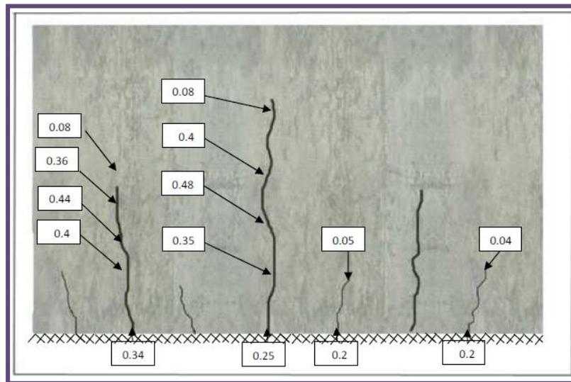
**Fig.1 Typical Cracks wWidths (mm) for Wall (Kheder 1997).**
