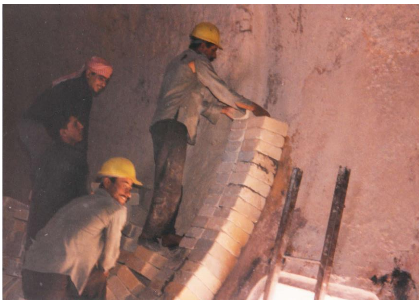
Fig 2 :Refractory Brick Re-building at Kufa Cement Factory (Kiln No.2).
