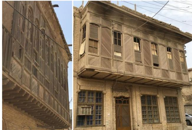
**Fig. 5:** Examples of Shanaseel base, one resting on wooden stands and the other on jack arch structure of iron and wood beams (newer) in the old city of Basra
