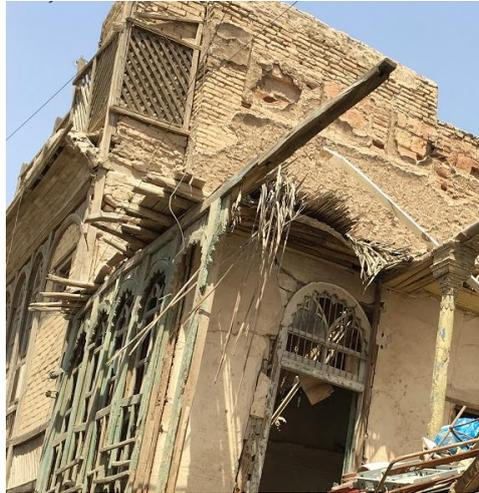
**Fig. 14:** A decayed roof showing the structural composition of the Jawi wooden ceiling of a Shanaseel building
