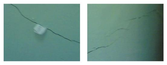
Fig (2) shows the cracks because the deflection
