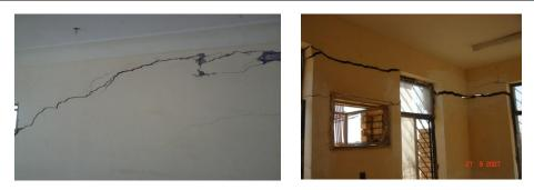
Fig (3) shows the cracks because the settlement
