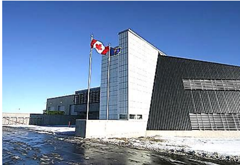
Figure 1. The front façade of this building is a transpired solar air heating system that heats the incoming ventilation air for the facility, [26]
