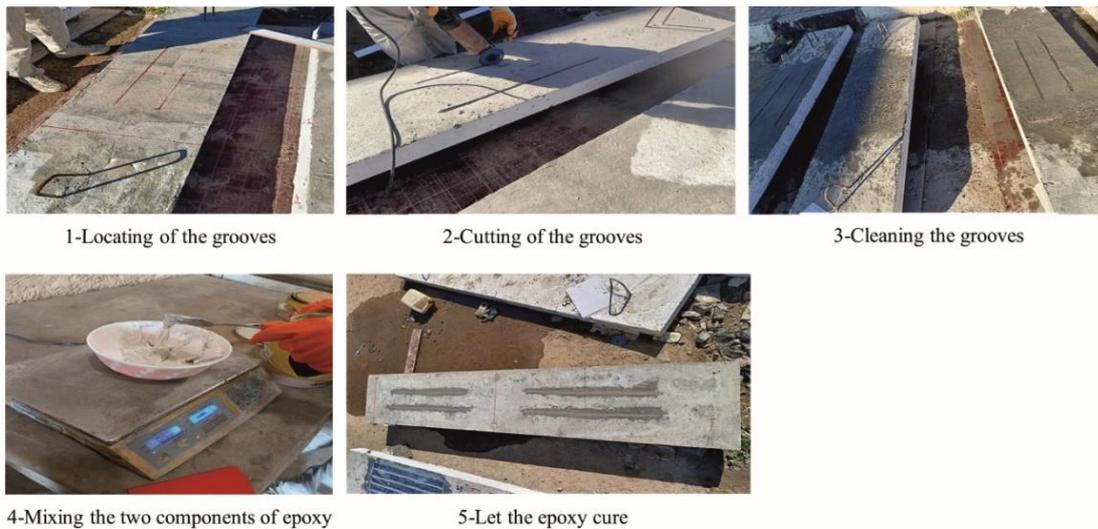
**Fig. 3. Steps of repairing the RC slabs with NSM CFRP bars.**
