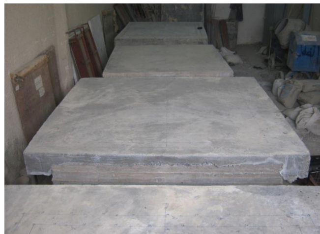
Plate (1): Reinforced Concrete Slabs.
