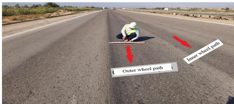
Fig. 3 Measurement of rut depth in the inner and outer wheel tracks of Express No.1 for Station 46+500 in Part R9/A.
