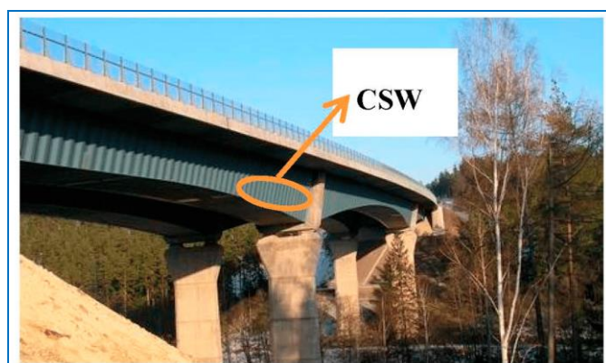
Fig. 1 Bridge constructed using girders with a corrugated steel web.
