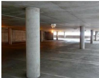
Figure 1. Flat plate concrete system [3].
