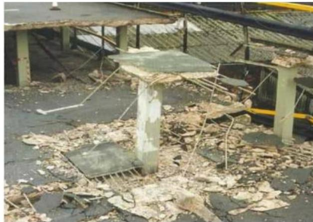
Figure-2 Common punching shear failure [4].
