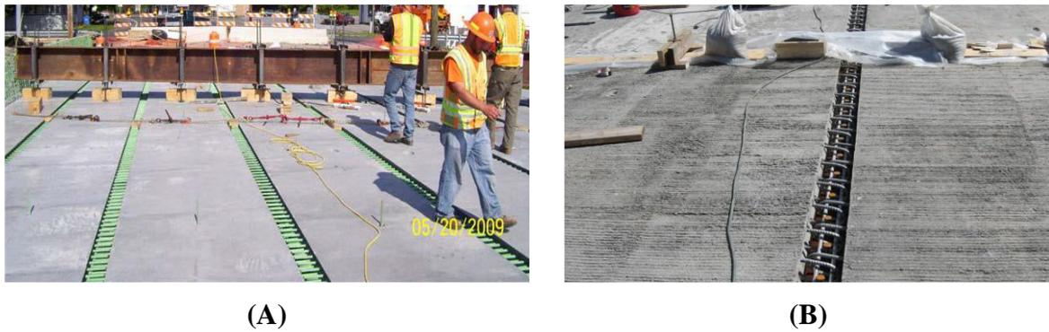
Figure 2 A) Longitudinal joint in route 31 bridge and B) Transverse joint in route 23 bridge [3].
