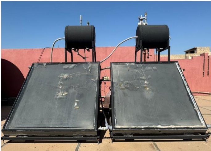
Fig. 2. Photograph of flat plate collector.
