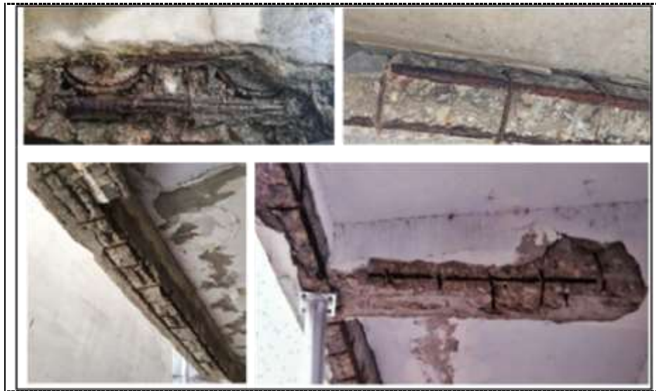
Fig. 1: Corrosion of steel bars in RC structures [14].
