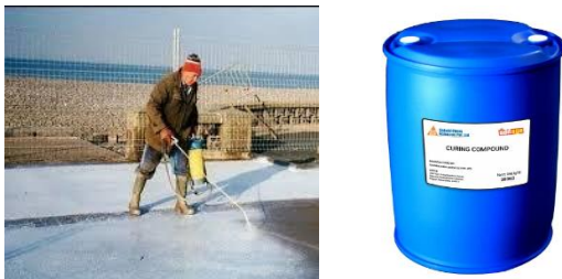
Figure 6. Chemical compound curing
