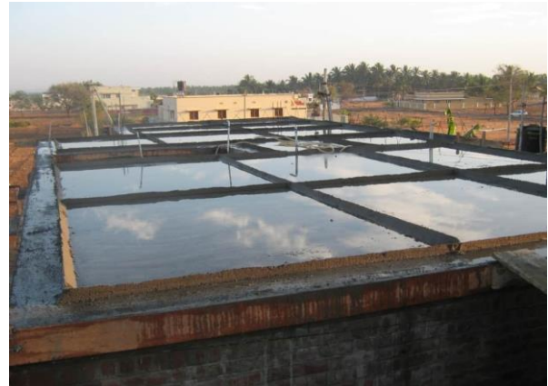
Figure 2. ponding concrete method
