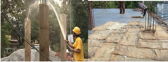
Figure 3. Covering concrete surfaces with hessian
