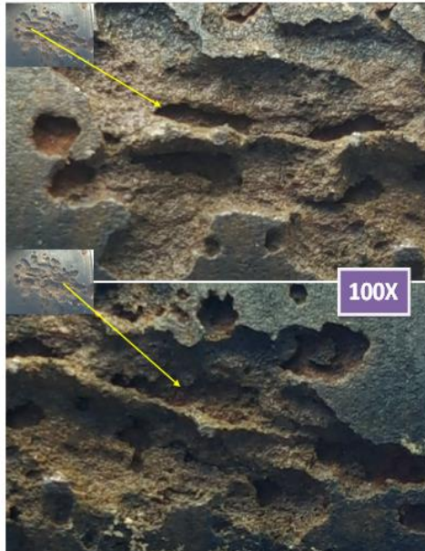
Figure (6) Corrosion effect on convex area of the specimen at the last day in January
