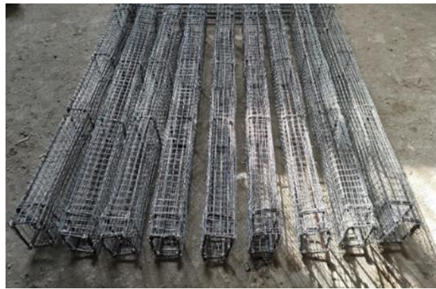
Fig. 5 Reinforcing steel for beams (FC)
