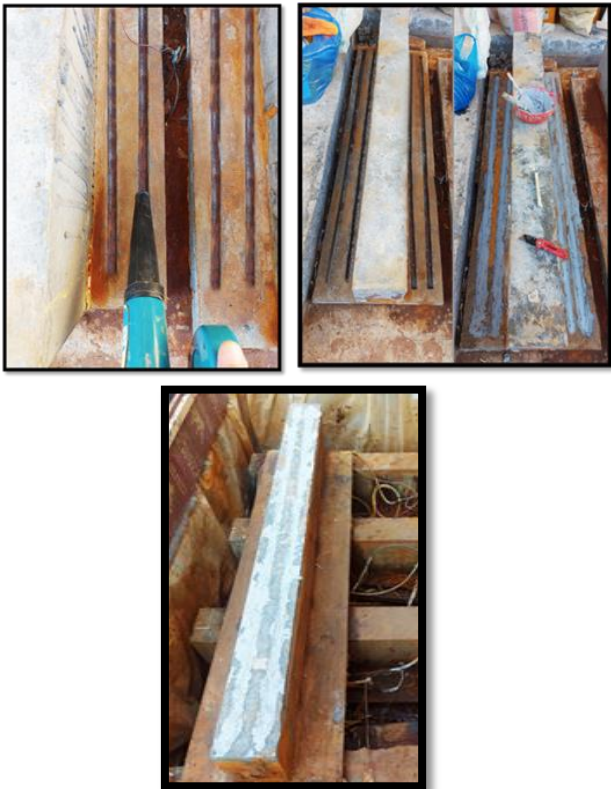
Figure 8 Implementing the NSM technology on corroded beams
