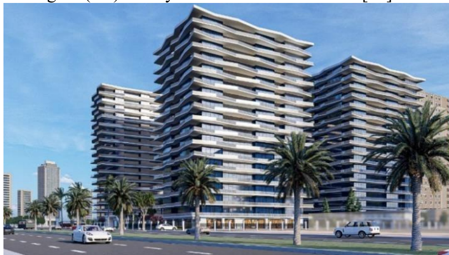
Figure (3.1) Wavey Avenue Towers. Source: [20]
